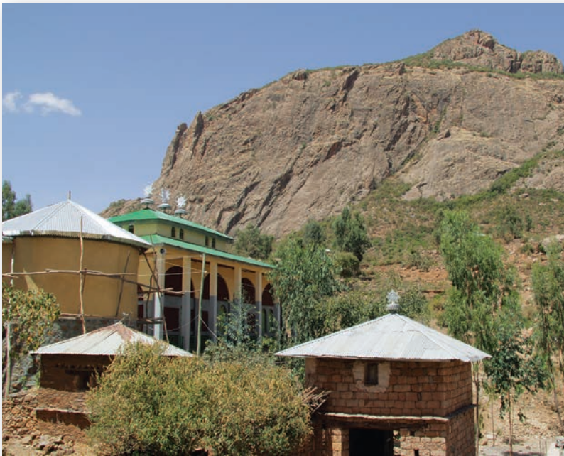
The Abba Garima Monastery resides high on a cliff near Adwa, in Northern Ethiopia, a highland area with a rugged topography. The large building on the left is the monastery church.
