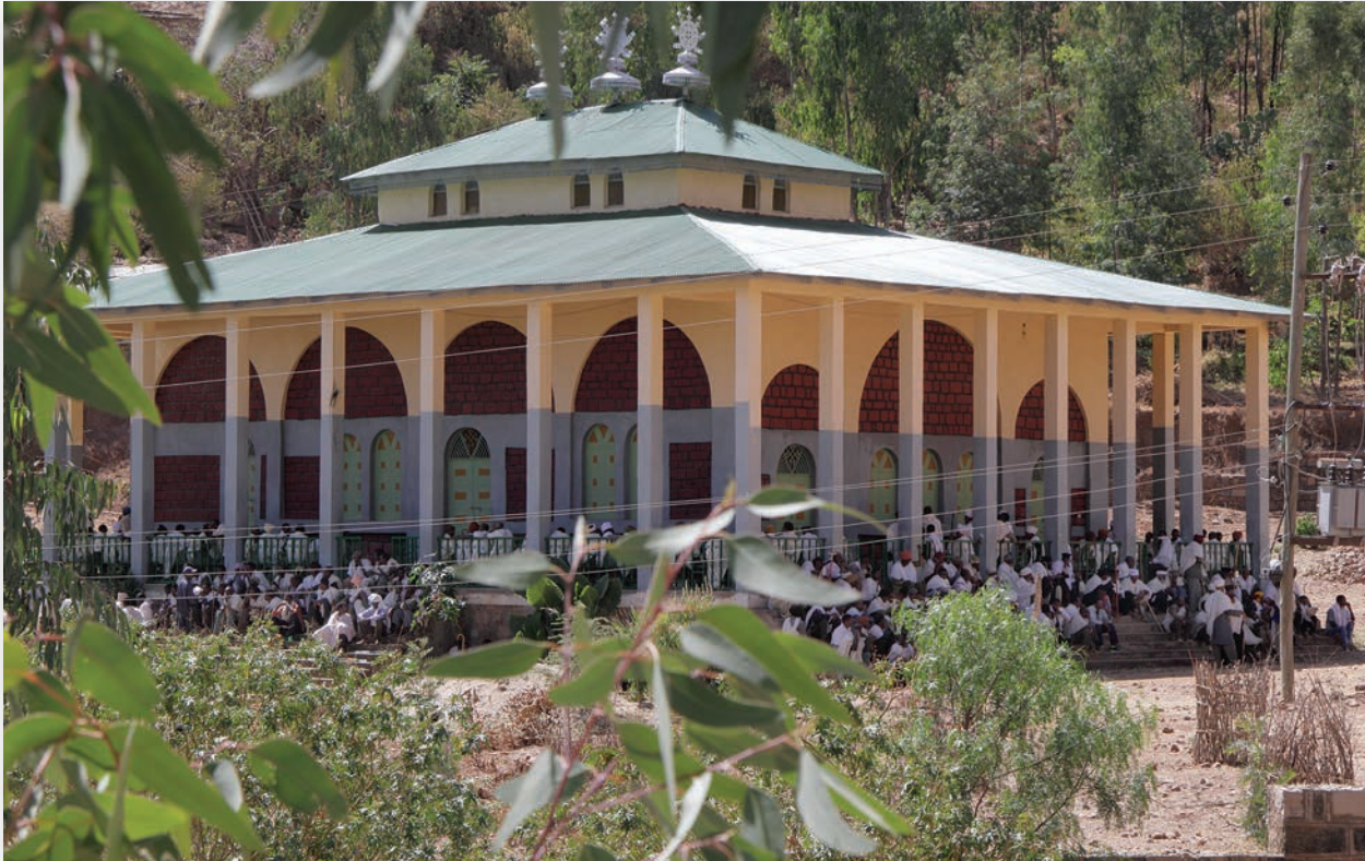
The church on the monastery grounds sits near the road and serves as the central meeting place for prayer and services. The monastery residence is further up the hill; no women are allowed in the residence. Here, parishioners gather in the shade after worship.
