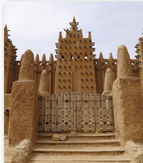
LEFT: The great Mosque of Djenné, Mali, is a UNESCO World Heritage Site. It is the largest mudbrick structure in the world.
